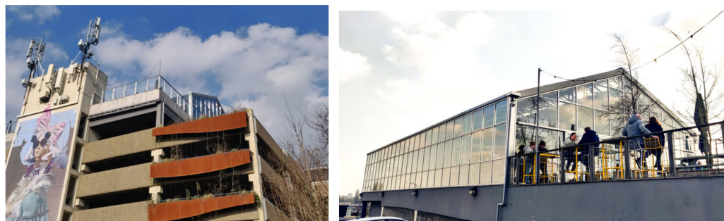
Figure 11. De Dakkas. The restaurant and event hall greenhouse on the roof level of the parking building, Haarlem. Credits: L. Zaffi, M. D'Ostuni.
