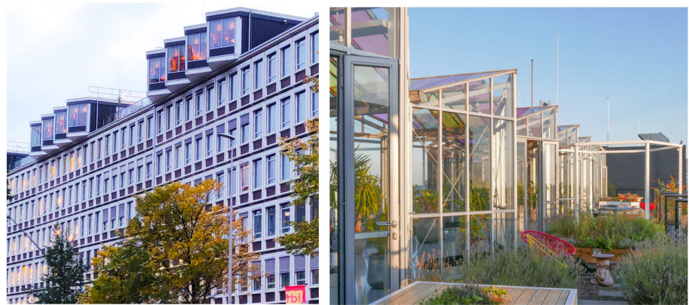
Figure 9. Zoku. The addition of greenhouses on the rooftop of the anonymous modernist-style block in Amsterdam. Credits: L. Zaffi, M. D'Ostuni.
