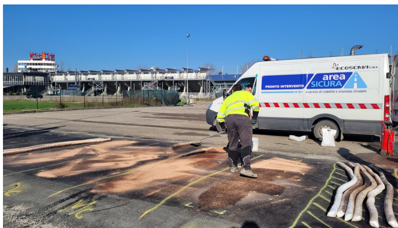
Figure 6. Image of pavement sweeping site.
