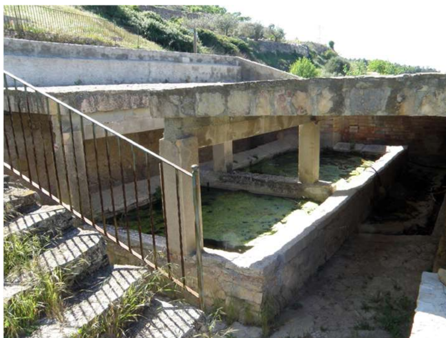
Figure 13. Wash place next to the Font Vella spring (la Figuera). This structure was restored in recent times, with repairs to the masonry wash basins and stone scrubbing decks. Photo credit: R. Pascual.
