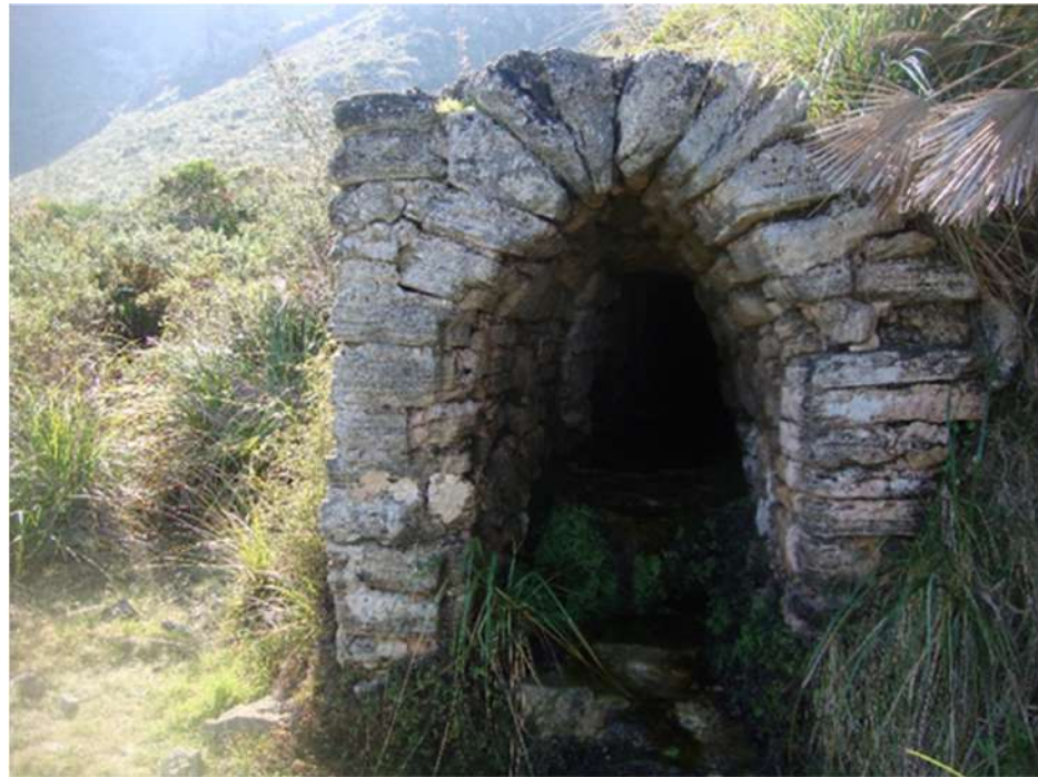
Figure 15. Fonts des Tions , spring-flow tunnel located in Artà mountains, east Mallorca. Photo credit: P.F. Castro.
