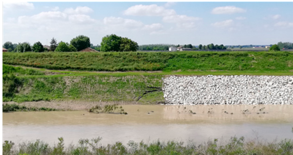
Figure 4. Deep-rooted plant planted on the Panaro River embankment (left side).
