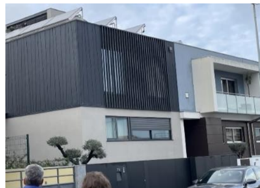
Figure 2. View of the demonstrator building.
