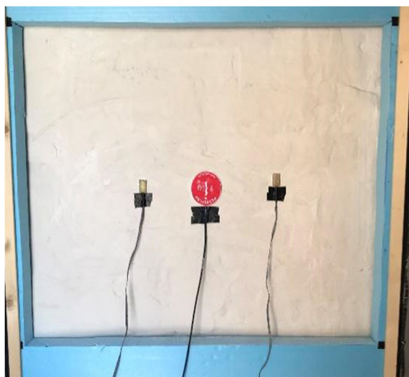
FIGURE 3 Sample panel with heat flow meter and temperature sensors mounted for the thermal tests.
