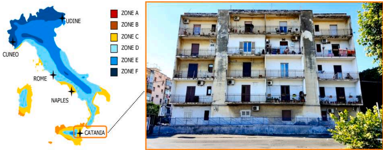
Fig. 1. The climatic zone and pilot building under study.
