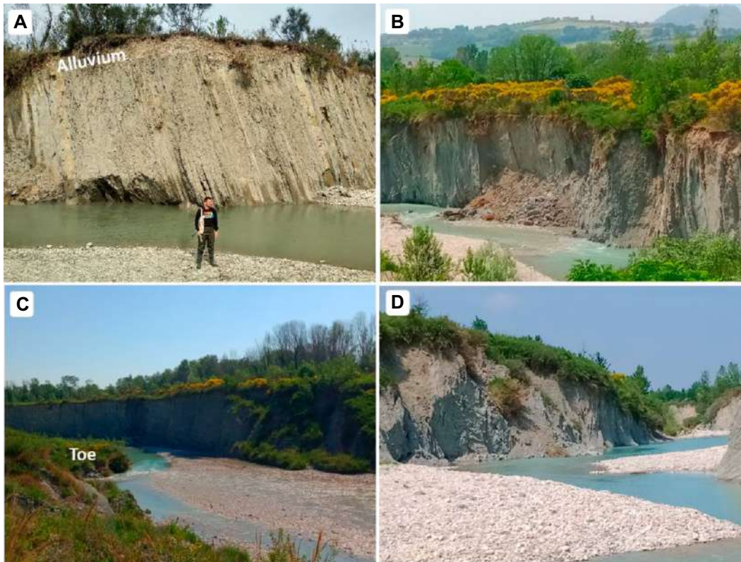
Figure 11. (A) Example of alluvium thickness (i.e., < 1 m) over sub-vertical pelitic layers (reach 15). Note the incipient slope undercutting at the base. (B) Talus deposit associated with a recent wall collapse (reach 16). (C) Toe of a rotational slide (left) moving to the right and deflecting water flow to the opposite canyon side, which consequently promotes undercutting (reach 15). (D) Point bars in a meandering stretch of the canyon (reach 16). Note the recent instability on the front wall induced by flow deflection at point bar.
