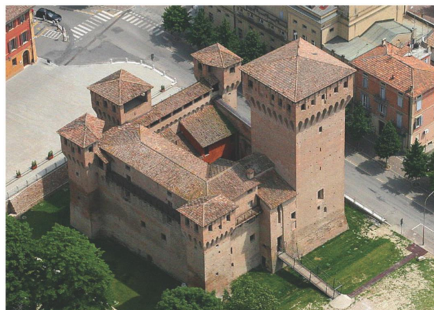
Figure 1. Bird-view from south-west of the fortress before the earthquake.
