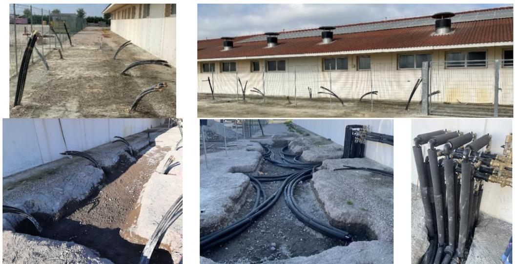
**Figure 17.** Realization of the BTES system: installation of the 8 BHEs and pipe connections.
