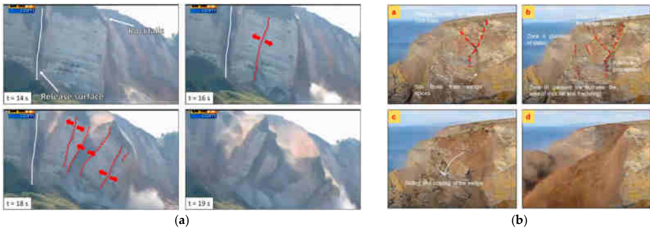
Figure 11. Examples of type 4 slope damage: (a) Frames extracted from an online video of the toppling failure of a sea cliff in France (from https://www.youtube.com/watch?v=gvSe27Ht-NY , accessed on 2 December 2022). The white line shows the existing release surface at the rear of the unstable block. Red, dashed lines mark fractures that opened during the displacement of the landslide, which did not affect the detachment or the kinematics of the landslide. At t = 16 s, note the rockfalls preceding the detachment of the block, enhancing its kinematic freedom. (b) Frame video analysis showing the development of slope damage during the displacement of a landslide that affected the Hell’s Mouth cliff (Cornwall, UK, from [159]).
