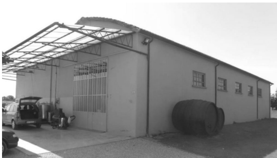
Fig. 1. Case study building
