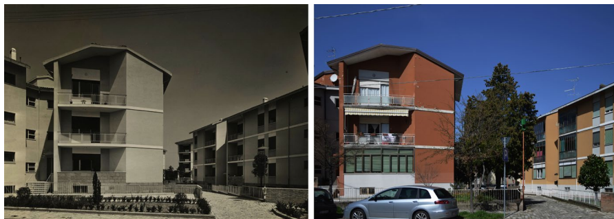
Fig. 14.2 – Find the differences: the typical transformation of multi-family buildings in less than 50 years. More than ten differences emerge clearly, such as the glazing closing loggias, and many more have been performed inside.
