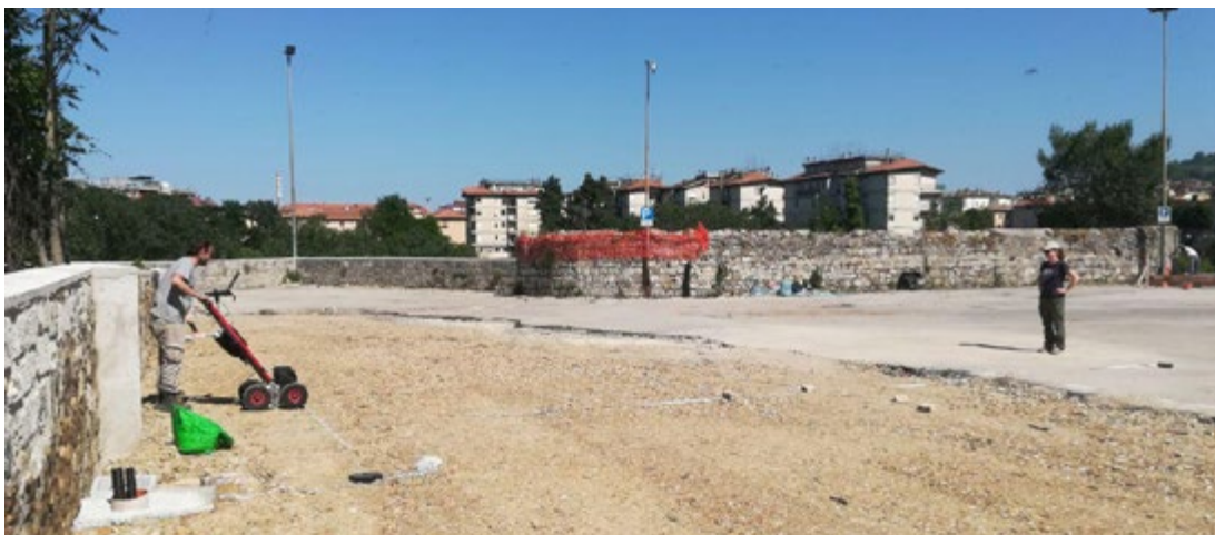
Fig. 5. Survey on field using Ground Penetrating Radar (GPR).
