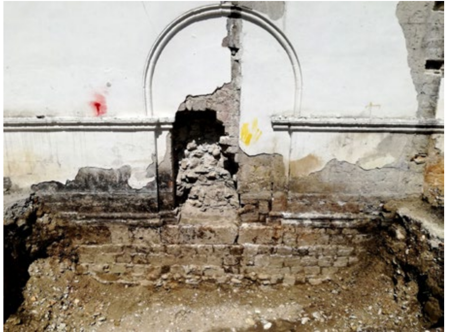
Fig. 16. Side façade E of the church.
