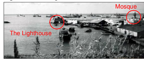
Fig. 13: Anchorage Area, North Border.
