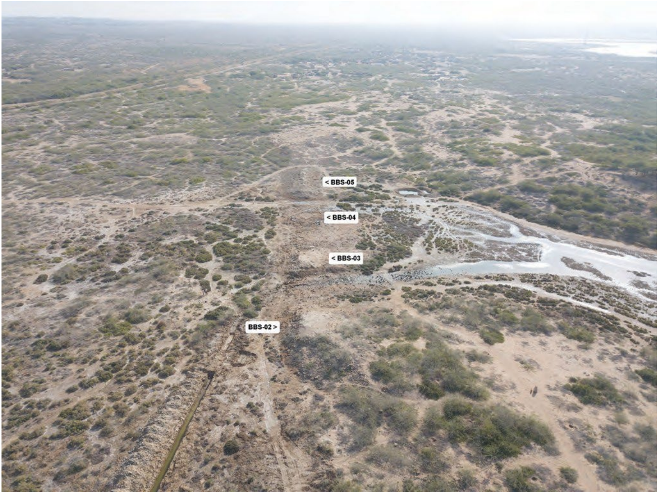
Figure 7. The ancient bridge after its cleaning; 2018 aerial picture, from West (operator: A. Tilia).
