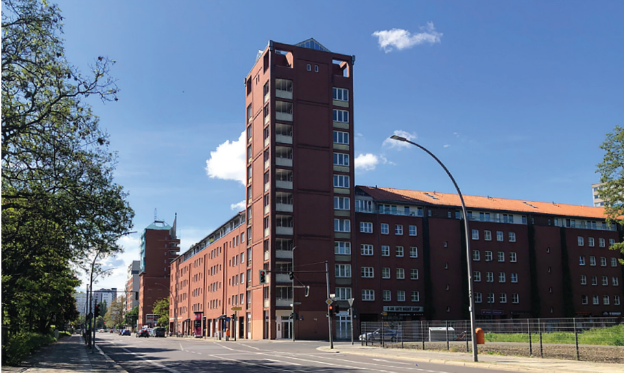
Fig.7: Block 9 (1985-1988). Top: View from Wilhelmstraße of the tower designed by Grupo 2C, with Pietro Derossi's tower in the background. Right: floor-plan typologies of the IBA buildings in the block.
