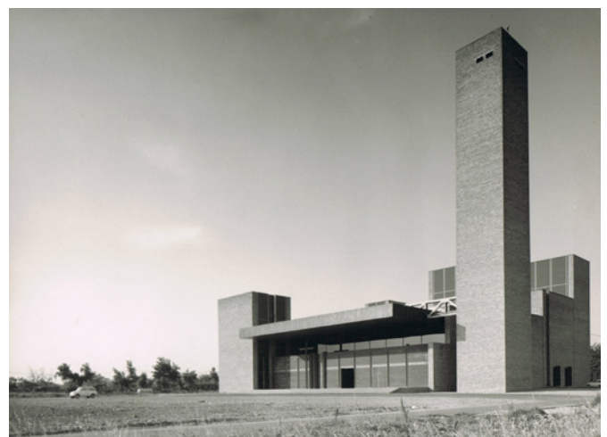
Fig. 4. The church during the last phases of the construction works.
