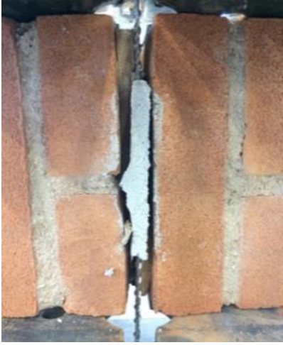
Failure mode A: splitting of the masonry wallette
