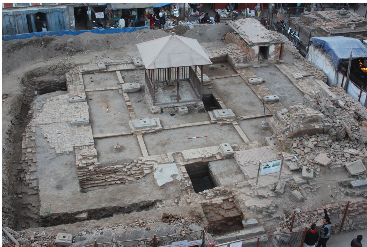
Fig. 9 Nine-celled mandala formed through brick-piers, foundation wall and cross-walls uncovered during archaeological assessments at the Kasthamandap
