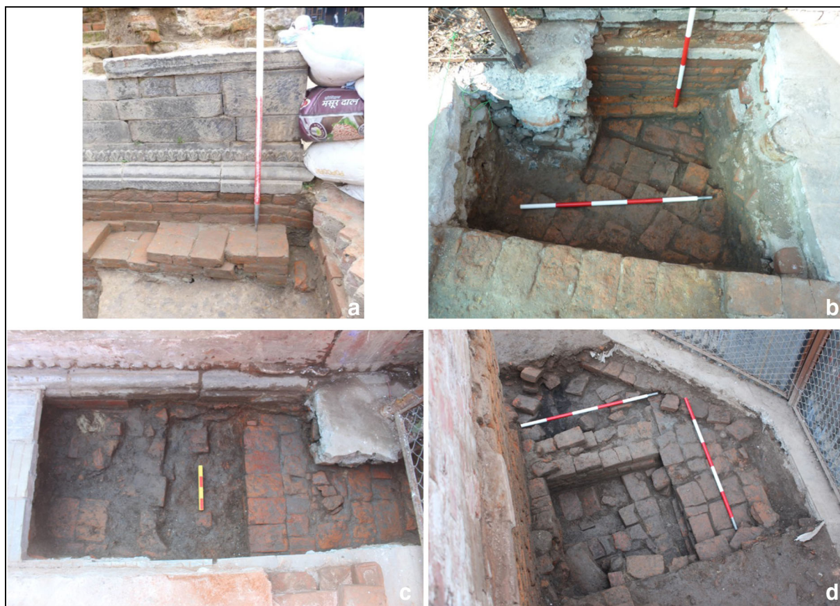
Fig. 6 The current footprint of the Vatsala Temple in Bhaktapur overlaying and overhanging an earlier brick foundation (a); a large brick wall on a differing alignment running under the plinths of the
