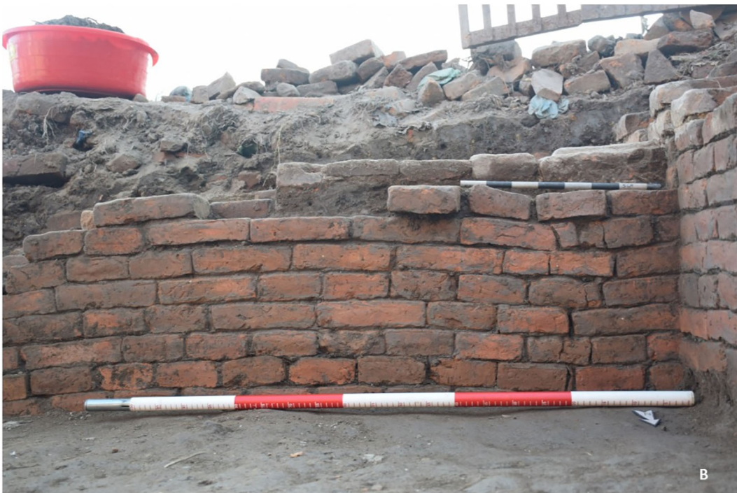
Fig. 10 Vertical cracks identified below a double saddle stone in the foundations of the Kasthamandap (a) and below a saddle stone in the foundations of the Gurujyu Sattal, Pashupati (b)
