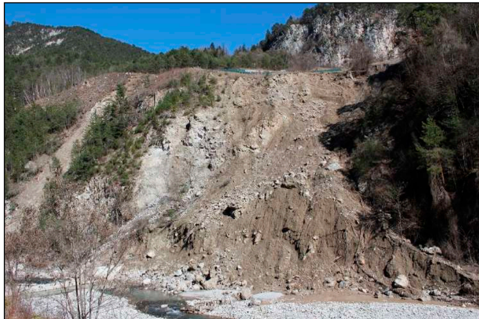
Figure 10. Frontal view of the landslide showing the complex composition of the soil involved.
