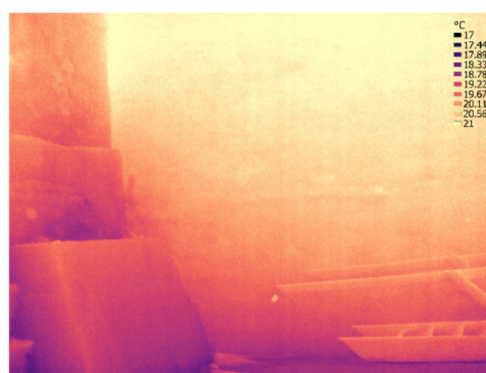
Figure 9: Thermal image of the interior south wall.
