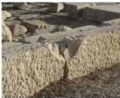
Figure 1. Stone plinths and pedestals in Pasargadae world heritage site (Fars province, Iran) in need of repointing with compatible restorative materials.
