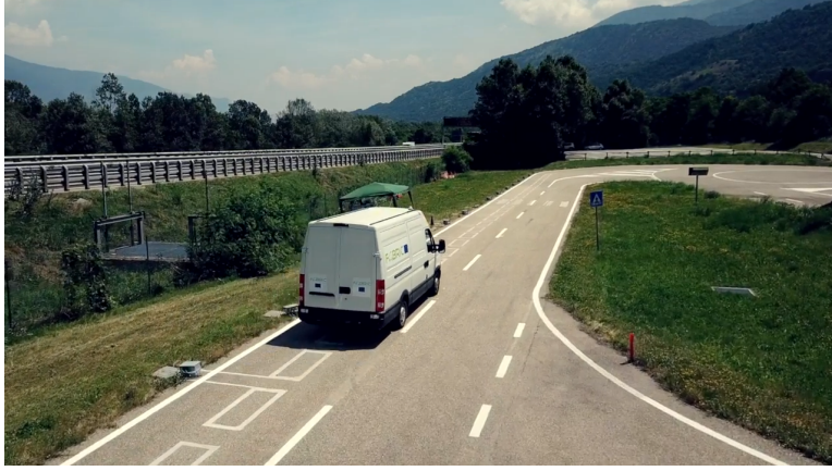
Figure 4: Picture of the PoliTO CWD system. In the picture are visible the shape of the transmitter coils embedded in the road pavement, the boxes containing the DC/AC converters placed outside their manholes, the equipped vehicle.
