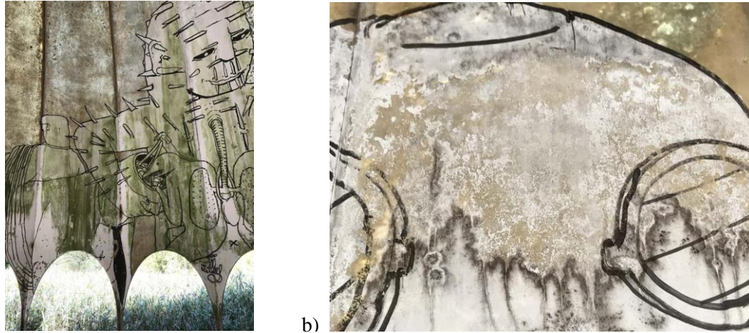
Fig. 13 a) Green patina covering the white paint in the northern vaults; b) dark stains on the paint in the southern vaults (the pulverization of the white paint can be noticed).
