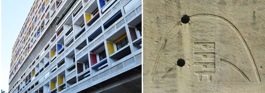
Fig. 2. Unité d’Habitation de Marseille, Le Corbusier. Main façade and detail of the sun path scheme drawn on a bench in concrete located in the external courtyard (C. Mazzoli, 2017)
