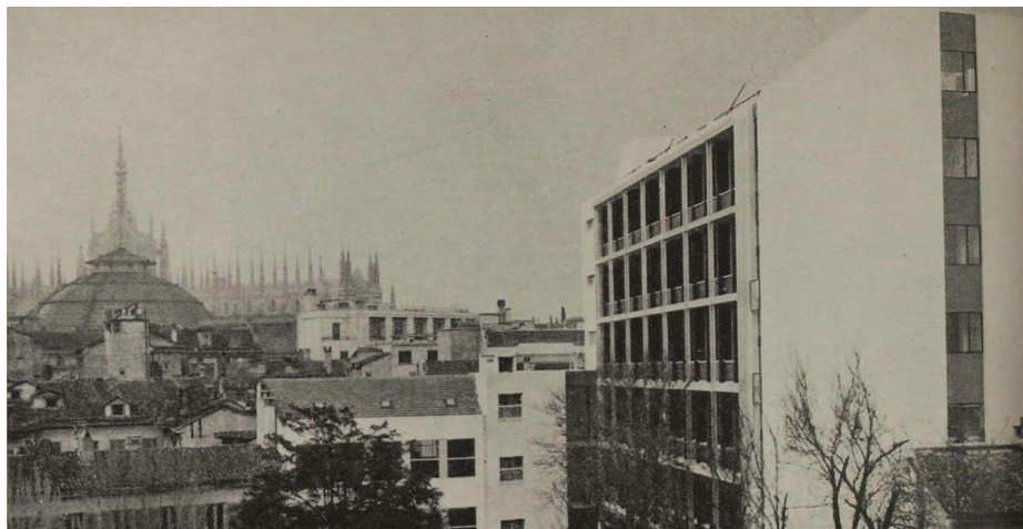
Fig. 11. Courtyard elevation with the view of the dome of Milan Cathedral on the background (source: Notizie Olivetti, n. 21, novembre, 1954)
