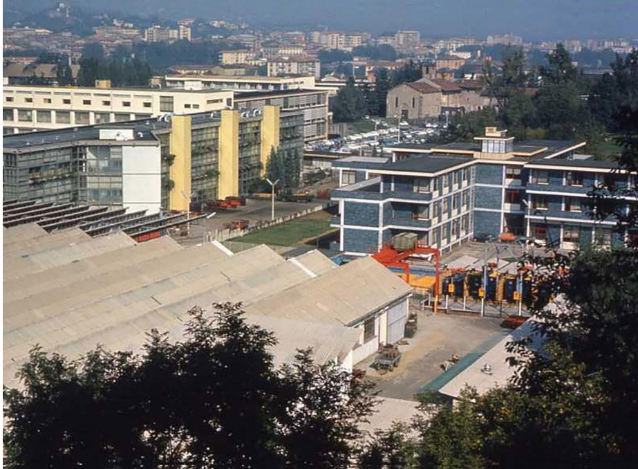
Fig. 8. The Center for Studies and Experiences built in 1954-1955 and designed by Eduardo Vittoria, its blue covering in ceramic tiles is clearly visible together with the yellow one of the New ICO towers (source: Associazione Archivio Storico Olivetti, Ivrea – Italy).
