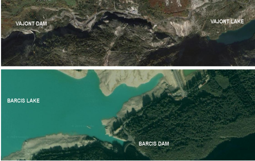
Figure 9. Aerial views of Vajont Dam and Barcis Dam (Google Earth).
