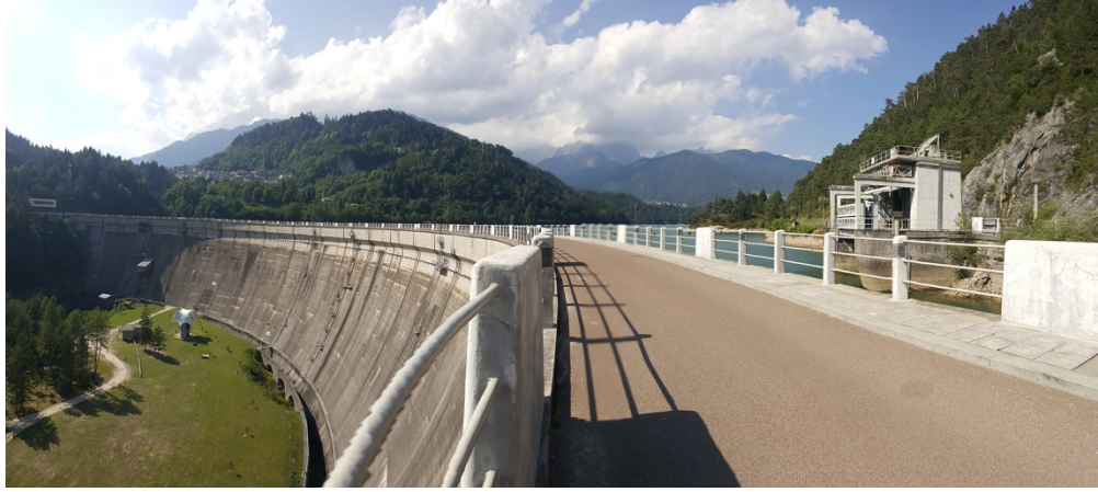
Figure 4. The dam and the intake structure of Pieve di Cadore (photo taken by the authors on 11.08.2019).
