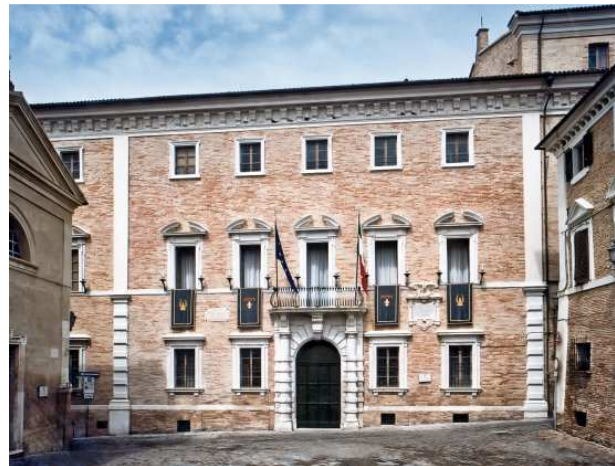
Figure 2: Campana Palace, Osimo. View of the main façade from Dante Alighieri Square.
