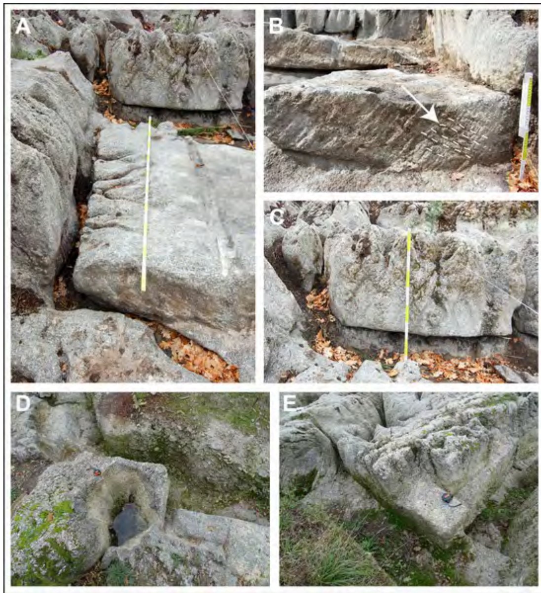
Fig. 7. Signs of excavation in the quarry: A. The straight groove on the floor of the third bench; B. Pick marks on the vertical wall of the quarry between the second and third bench (arrow highlights the area with the most evident grooves (dashed lines)); C. More or less defined block to be extracted (note the upper severely dissolved part), with the signs at its base where the wedges were inserted; D. Artificially enlarged and plastered cone-shaped pit and, to its right, a gypsum block partially prepared for extraction; E. Partially isolated gypsum block on the corner. Meter for scale.
