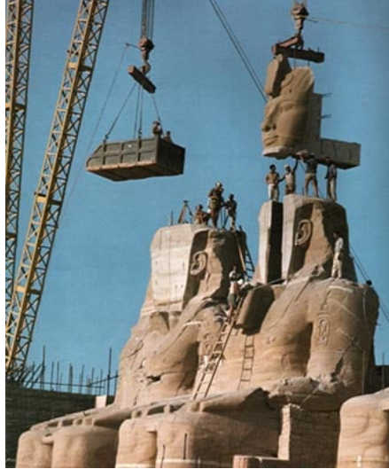
The reassembling of the statue of Ramses II at the Great Temple of Abu Simbel in 1967 after having been moved in order to save it from the Aswan dam flooding. (Wikimedia commons)
