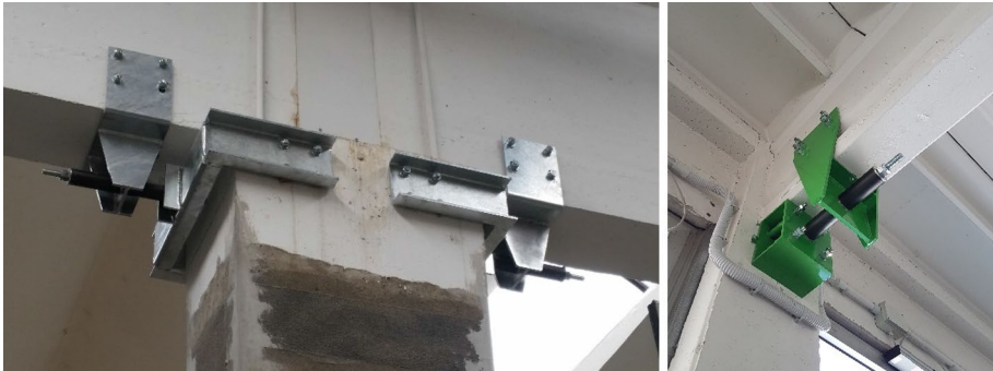
Fig. 2 Examples of beam-column connections with dissipative devices
