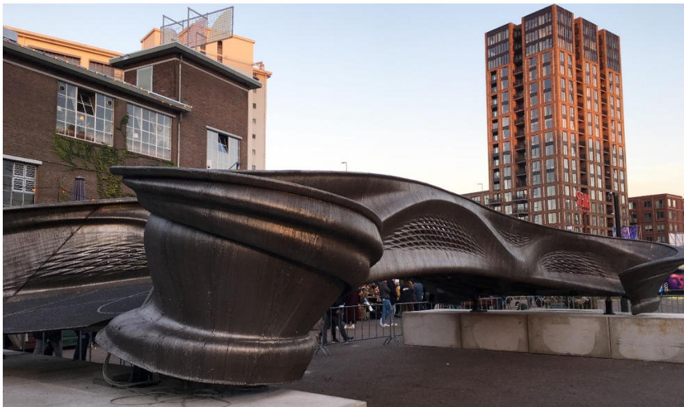
16 17 Figure 1: The MX3D Bridge [9]. 18
