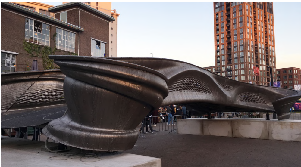
Figure 1: MX3D Bridge realized with WAAM process [16].
