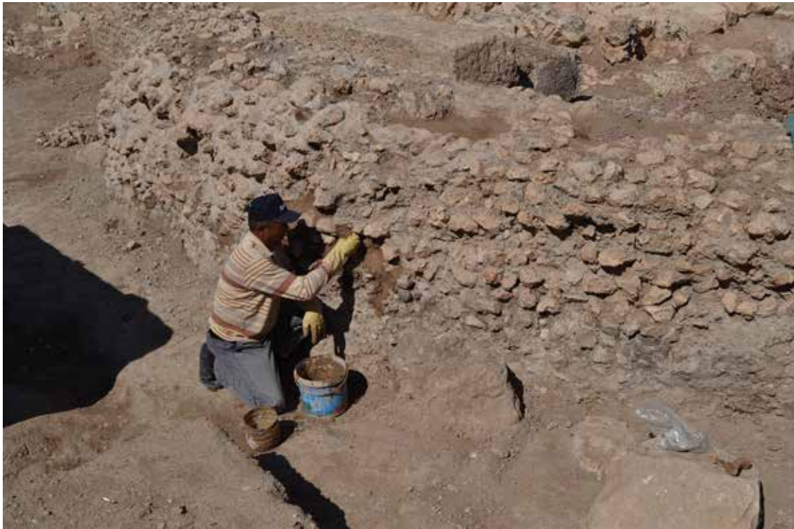
1. Conservation work of the Roman water conduit (phase 3).
