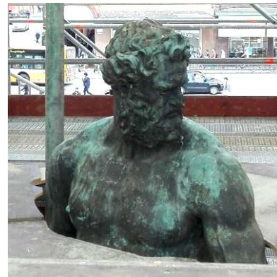
Figure 2. Neptune statue during the restoration works (detail).
