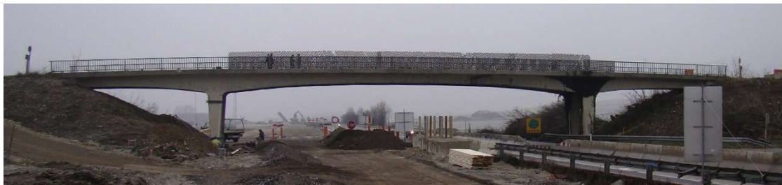
Fig. 4: View of the S101 Bridge [72].
