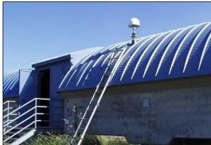
188 189 Figure 4. GNSS antenna mounted on the tunnel.
