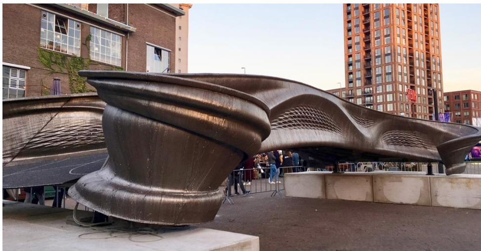
1 2 Figure 1: MX3D footbridge realized with WAM process and presented at the Dutch Design Week 2018 in Eindhoven [26]. 3
