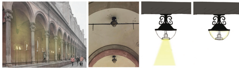
Figure 5: Via Zamboni porticos: display-cases for temporary exhibitions and historical lanterns subjected to conservative restoration.
