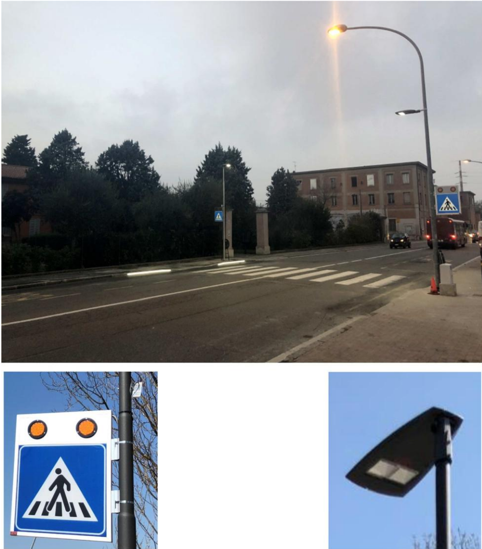
Fig. 3. Components of the integrated lighting-warning system: LED strips on both curbsides of the zebra crossing; backlit pedestrian crossing sign with flashing orange lights; dedicated lighting that enhanced the light power when the sensor detected a pedestrian. (For interpretation of the references to color in this figure legend, the reader is referred to the web version of this article.)
