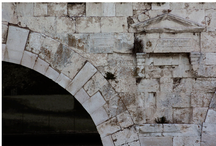
Fig. 17. Bridge of Augustus and Tiberius. A detail of the external wall casing. The lighter color ashlars are evidently the ones that were restored and have the mark of R 1976.
