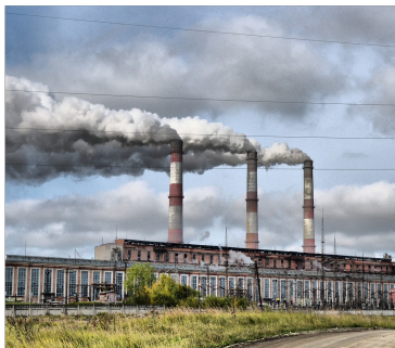
Figure 1: Smoke plumes from stacks.
