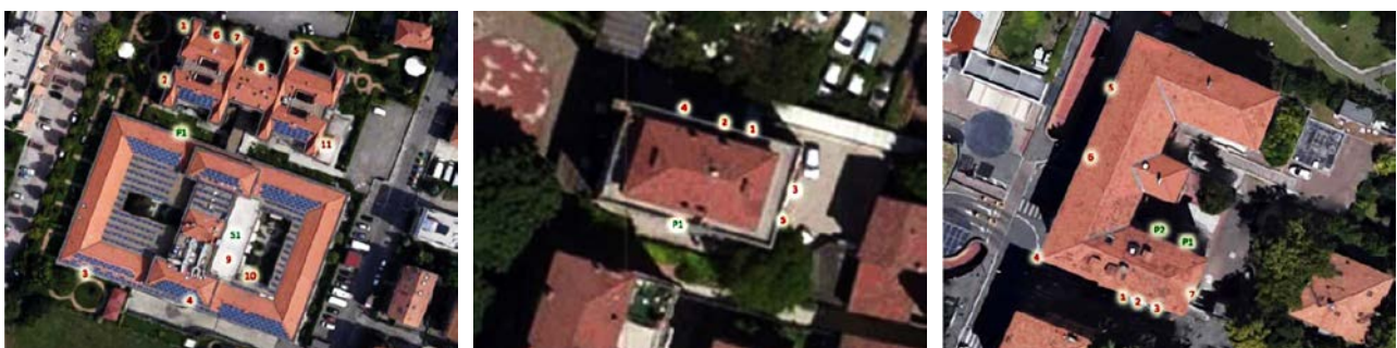
Fig. 2. Buildings No. 1, No. 2 and No. 3: aerial view and points of investigation.
