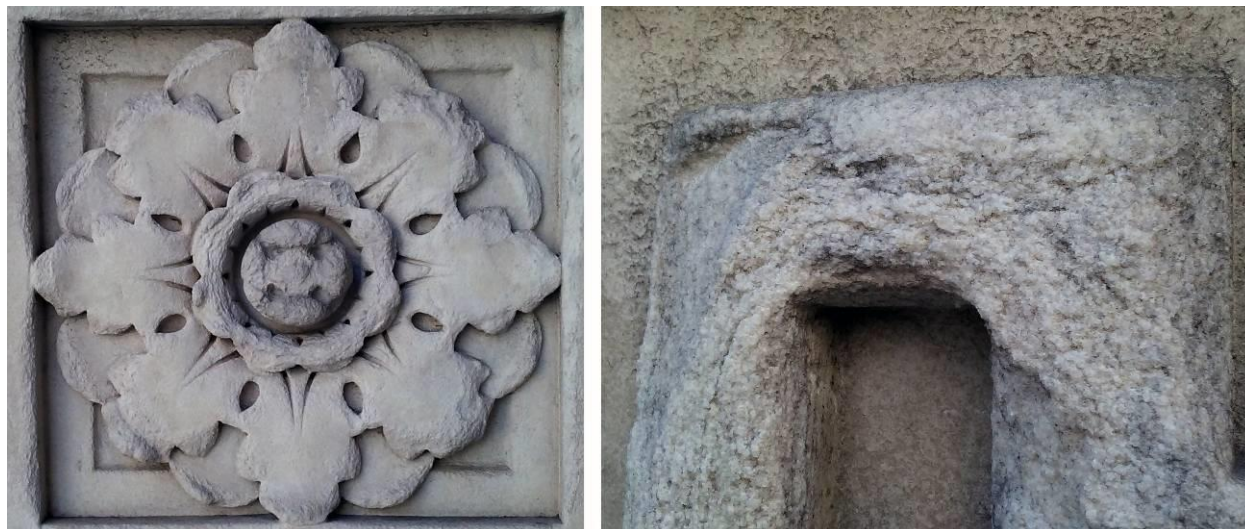
Figure 1. Examples of marble affected by sugaring in the New York Public Library (XIX cent).
