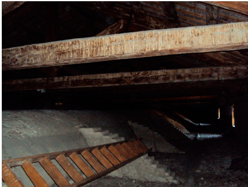
Figure 5. The attic on the top of the Library.
