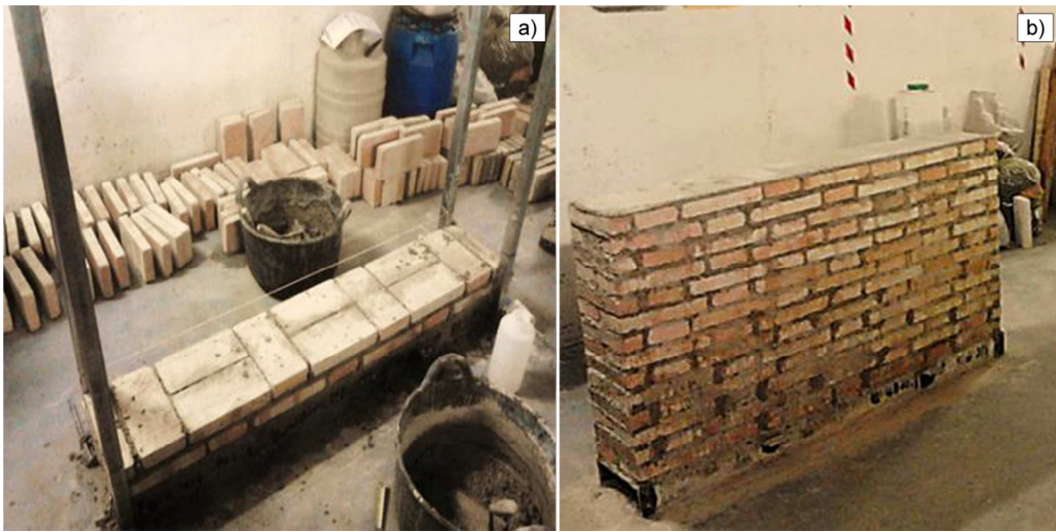
414 Figure 10 - Construction stage (a) and the wall at the end of the construction (b).
