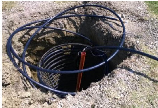
Fig. 2. The installation of the buried heat exchanger with the shape of a cylindrical basket whose performance is influenced by thermal properties of the soil.
