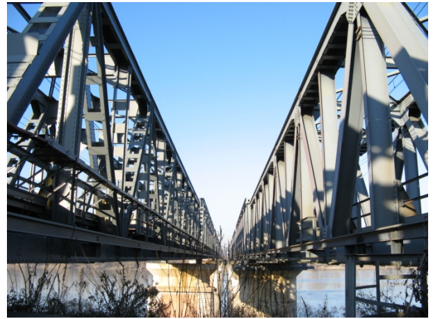
Figure 18 Case study No. 2: Old and new Pontelagoscuro truss-girder viaducts.
