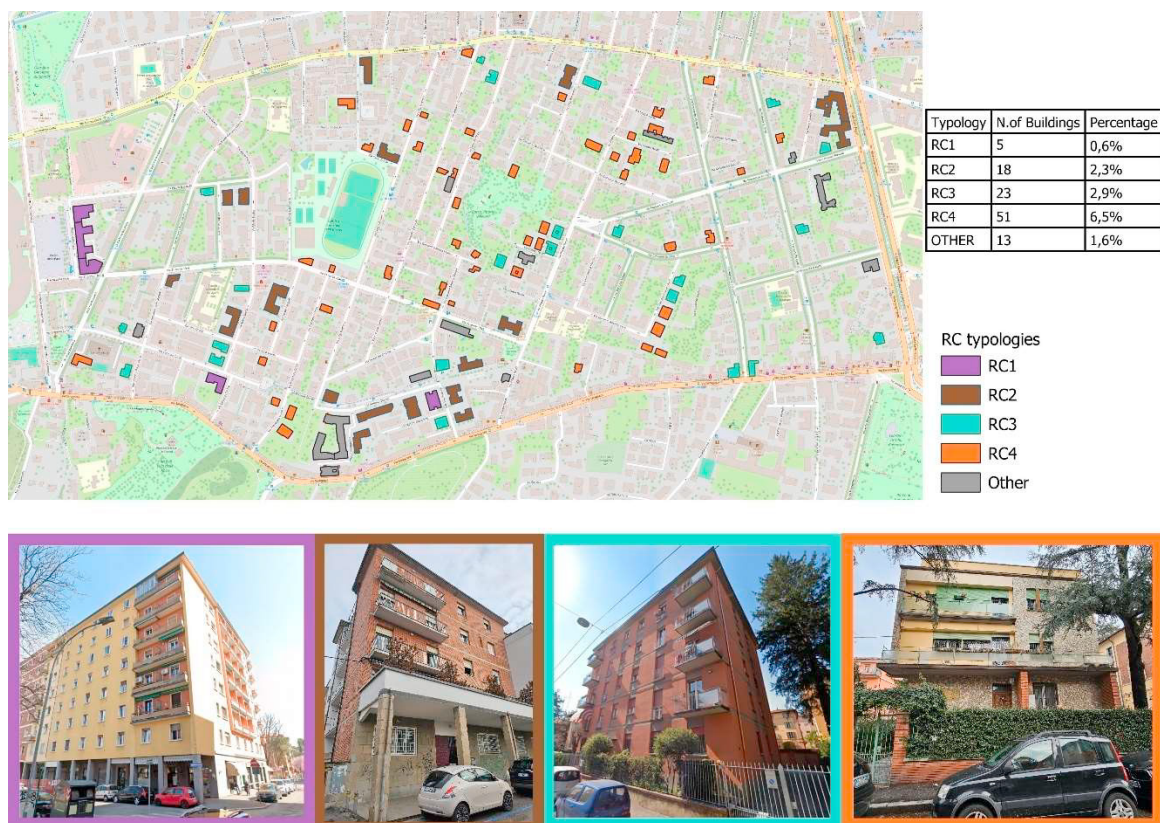
Fig. 6. RC building typologies in the Saragozza district (percentages are referred to the total number of residential buildings).
